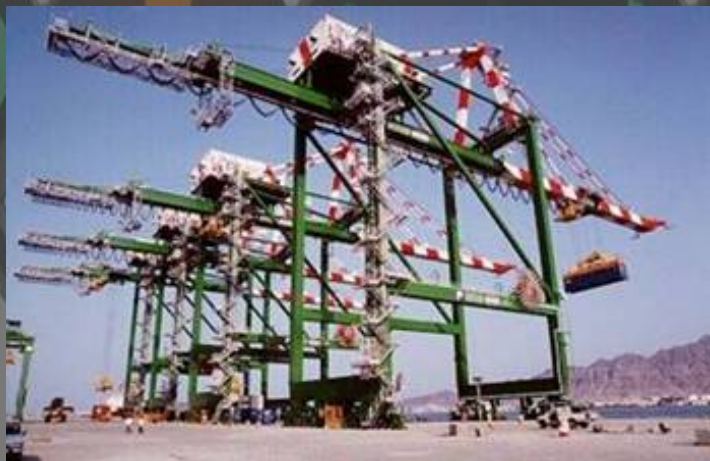
Aden container terminal
